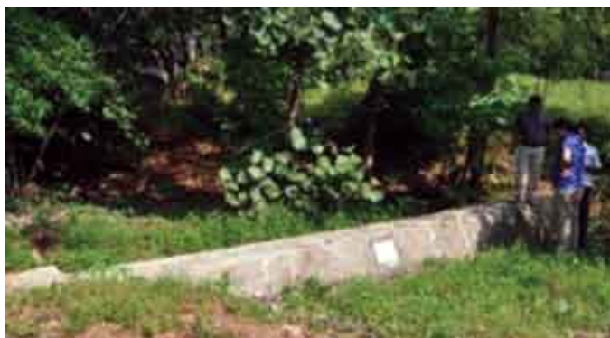
FIGURE 9 CHECK WALL IN GHATA VILLAGE
