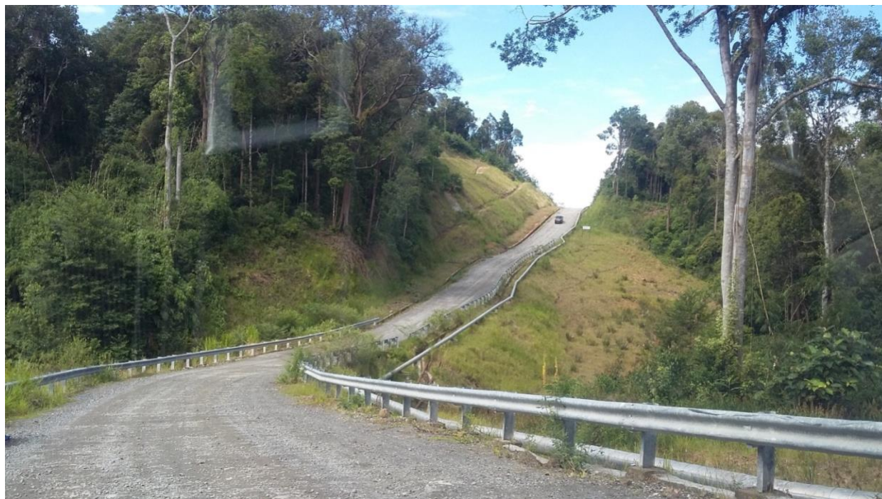
Figure 22. Sarulla project road showing wide cut-and-fill related clearing on either side of road for slope stabilization. Photo 2017 by E. Meijaard.
